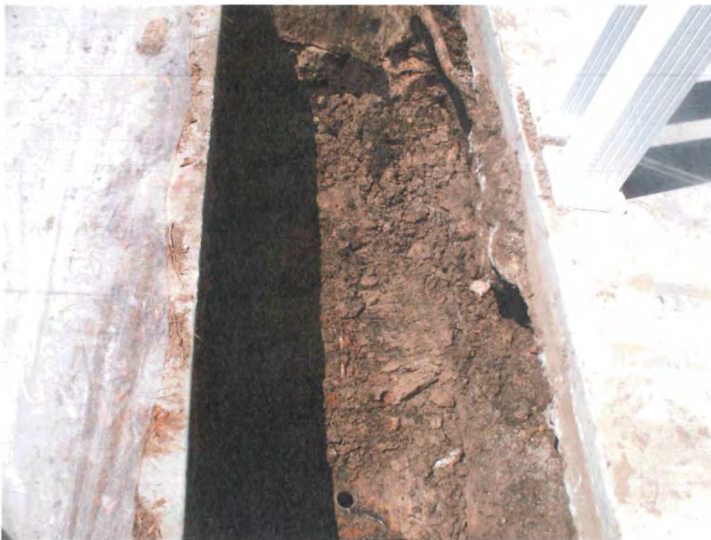
Picture 2: UST 332Ash excavation in progress.
